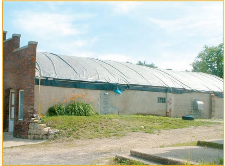
*Photo 5. The ratchet straps on the barrel ends holding down the roofing are not clearly visible. Although an extreme case, the materials that are visible are FM- and UL-approved. Specification of approved materials is not necessarily a good assurance of performance.*
