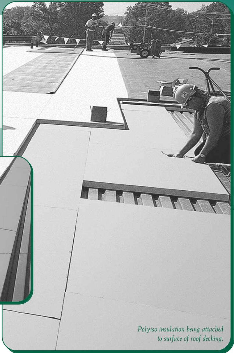
*Polyiso insulation being attached to surface of roof decking.*
