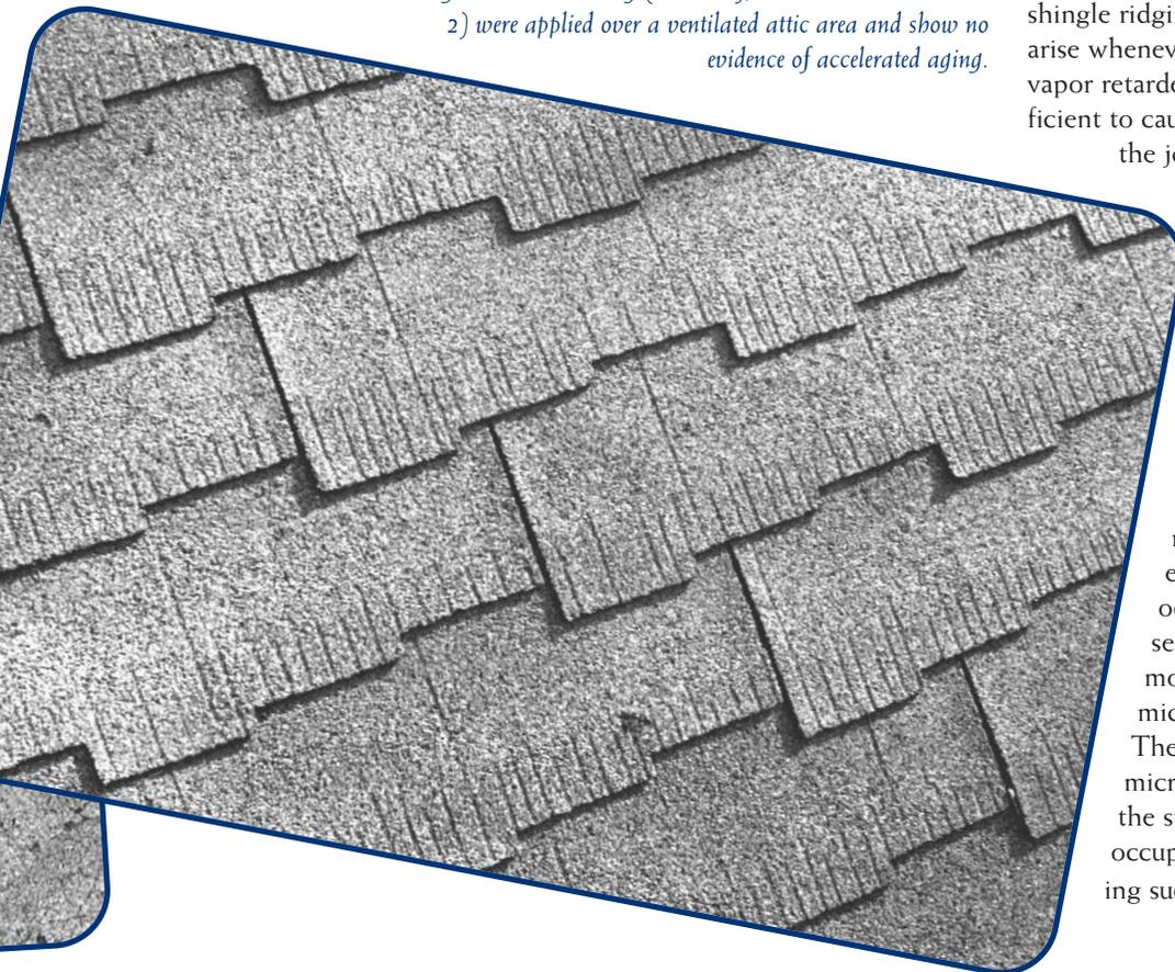
Another moisture-related issue is the potential for shingle ridging on new construction. This problem can arise whenever there is inadequate ventilation and no vapor retarder. Often the interior moisture drive is sufficient to cause buckling of the underlayment felt at the joints in the plywood decking and, consequently, the covering shingles. The resulting pattern of ridging often causes a concern to the owner.
