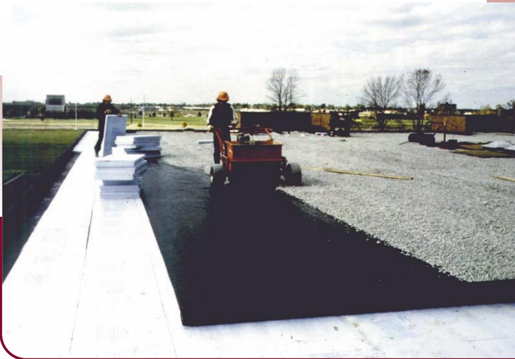
Figure I—Typical PMR system being installed.
