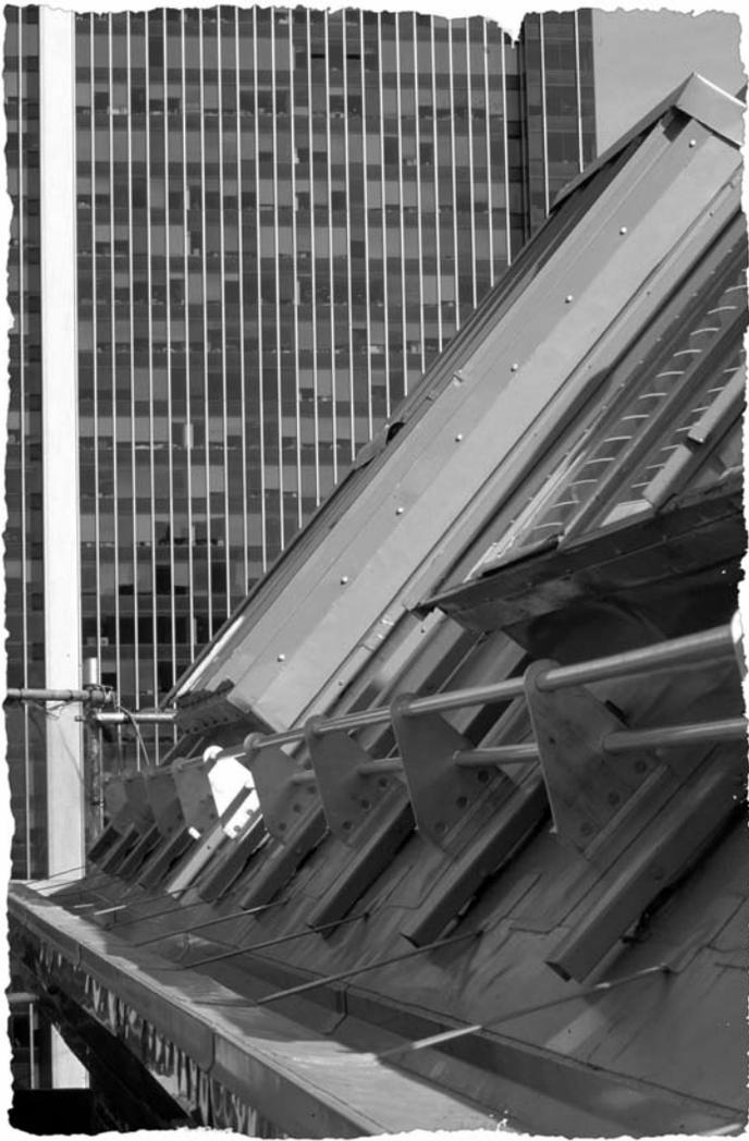
A detail of custom-manufactured skylights which perfectly match some 13 various-sized originals, as well as aluminum snowguard and flashing detail.
