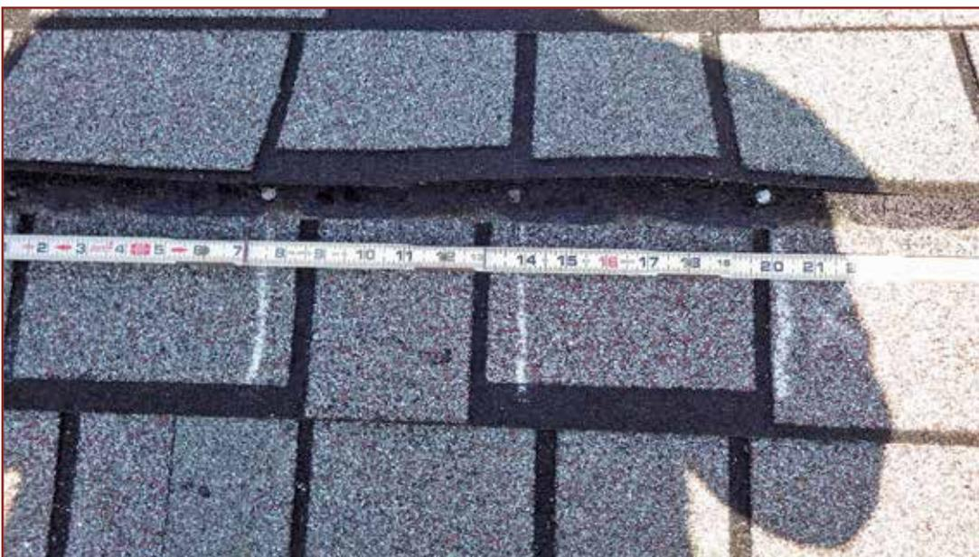
*Figure 4 – Forensic investigation of shingle installation documenting fastener placement.*
