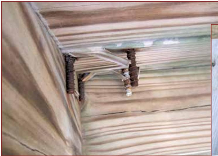
Figures 5 and 6 – Inadequate guardrail attachment.
