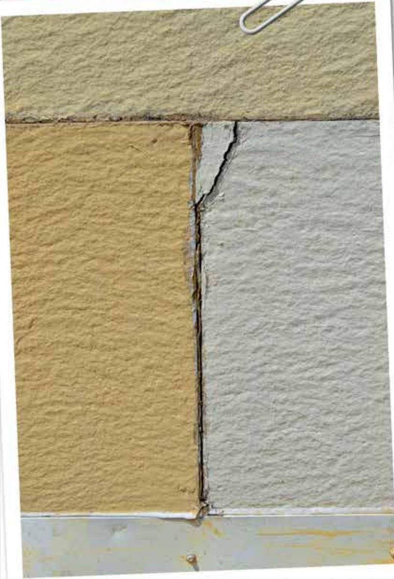
Figure 4 – Differential movement of the wall assembly resulted in excessive compression of the sealant joints and interferences between adjacent panels. Ultimately, this panel fractured as a result.
