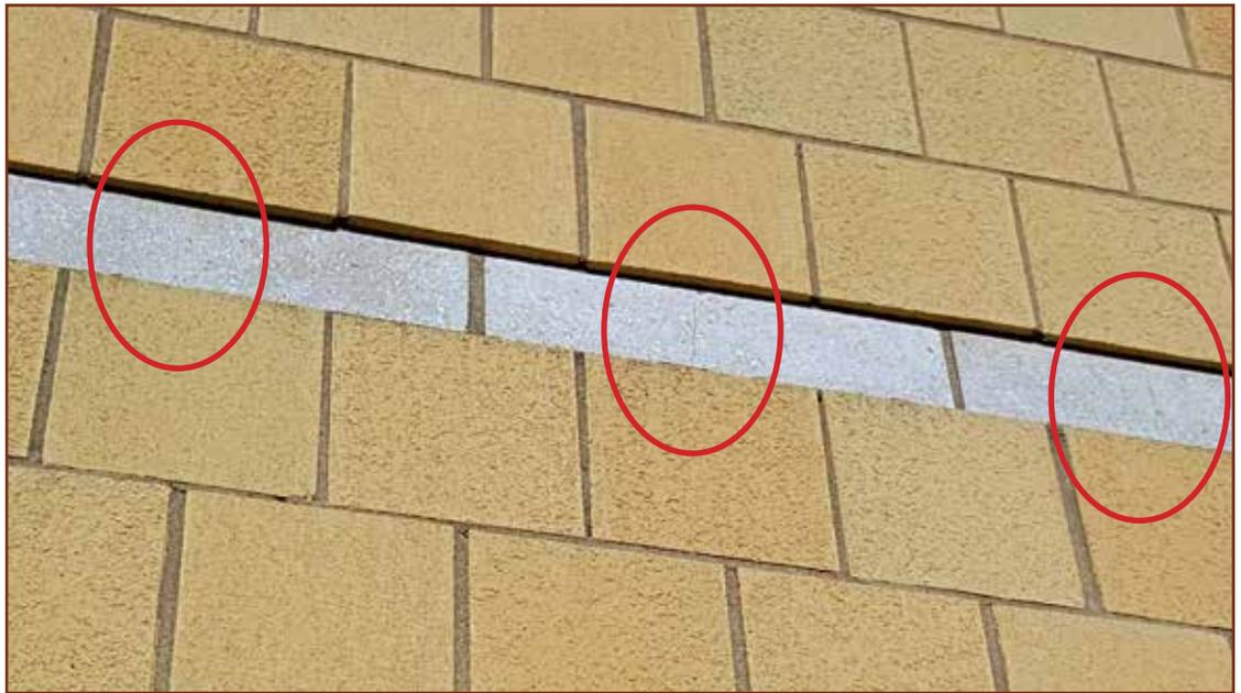
*Figure 8 – Approximately 80% of all CMU units are cracked in the accent bands on this large hospital project because of differential movement of the shrinking CMU band bonded to large expanses of clay brick veneer.*
