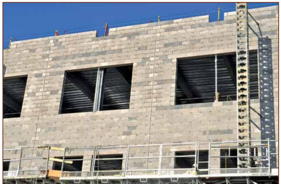
Figure 1 – Control joints properly located between openings.
