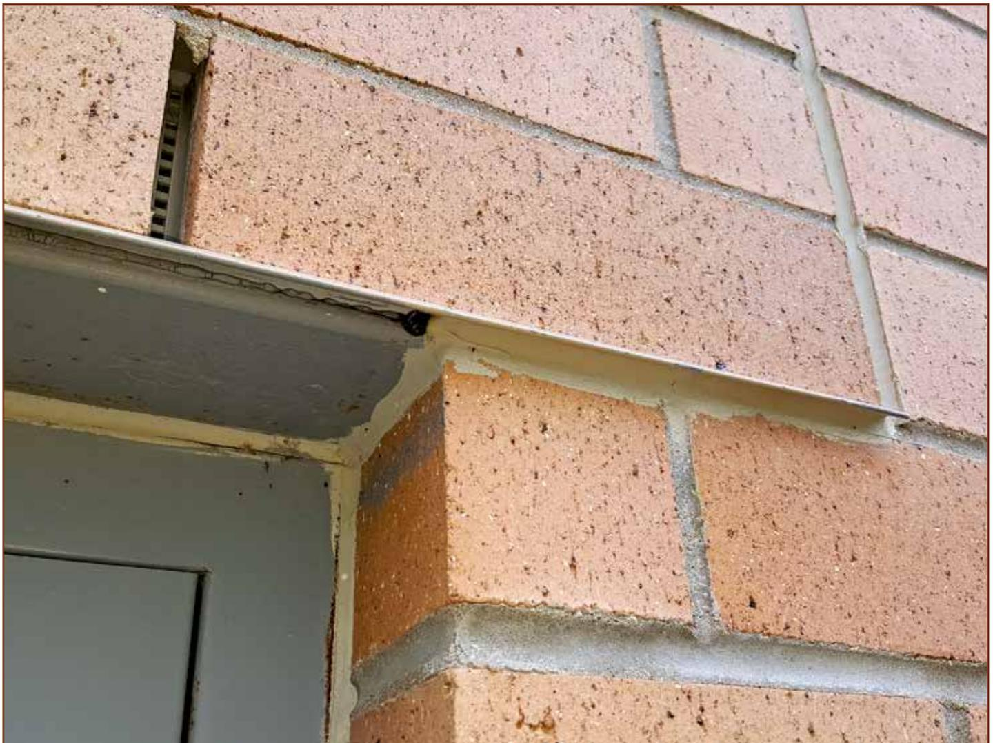
Figure 7 – Vertical movement joint properly located at the end of the beam bottom plate that supports the clay brick veneer at the door opening. Sealant properly installed under drip edge to prevent wind-driven rain penetration.
