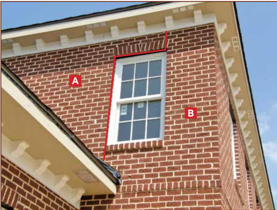
Figure 6 – The red line denotes location of a crack due to lack of isolation joint between elevation segments A and B, which have different bearing conditions. Segment A bears on steel, and segment B bears on the foundation below.
