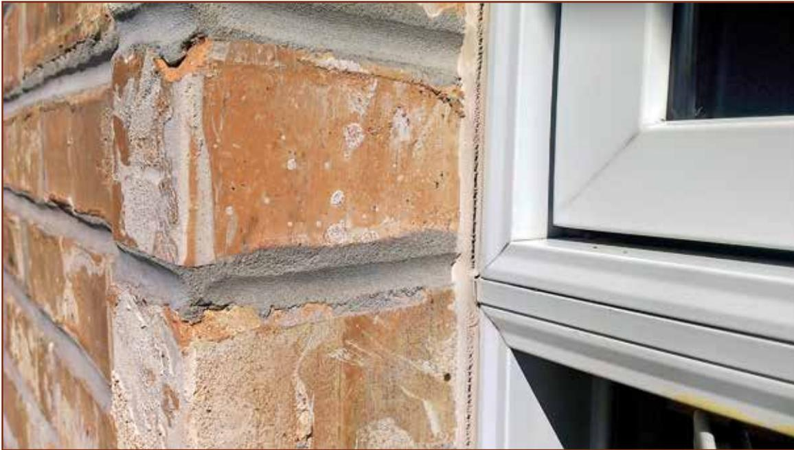
*Figure 9 – This sealant joint prematurely failed because there was no room to install a backer rod for a properly formed sealant joint. Designers should draw and dimension a gap on all four sides of windows.*
