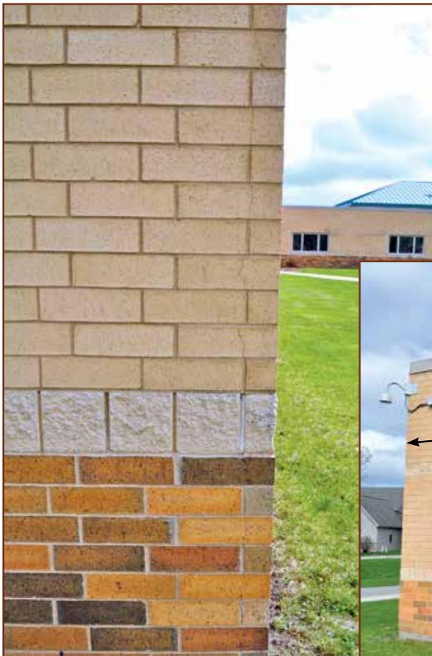
Figure 3B – Crack developed at the corner because veneer movement joints were spaced too far away from the corner on both sides.
