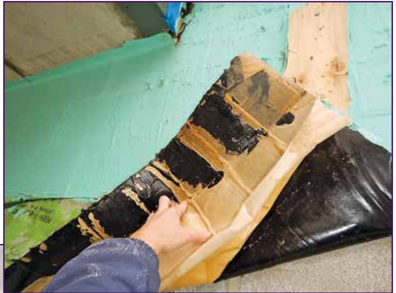
Figure 3 – Two months after seeing Figure 2, note the same TWF with intermittent loss of release paper and exposure to the elements, leaving self-adhesive or “sticky” side compromised to the extent that failure will occur.
