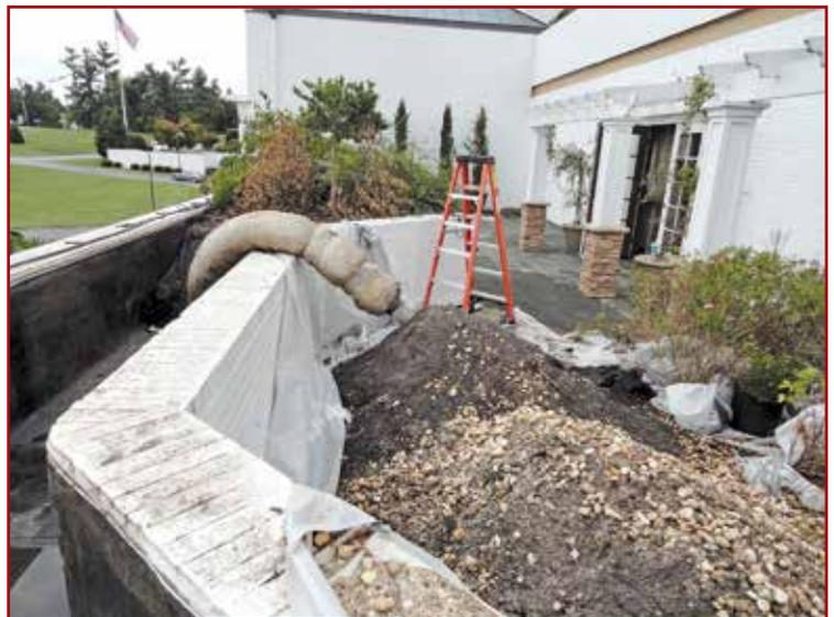
*Figure 2 – Chasing leaks in planted roofs can be tedious work. Mulch and organic fill may be the necessary environment to foster insect colonization; the invading creatures may also arrive on the various plantings being introduced.*
