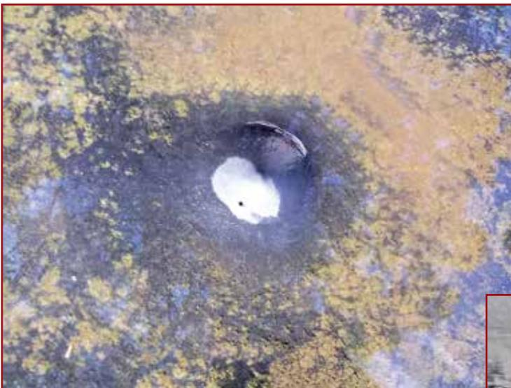
*Figure 6 – Although in near proximity, the tiny holes encountered here were not punctures from the nearby fastener head. The “tented” fasteners, however, may well provide the necessary underside space accommodation for the guilty insect to make the openings.*
