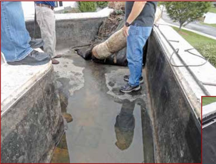
Figure 3A – This vessel incurred substantial cost, requiring removal of overburden where insect boreholes were eventually located.
