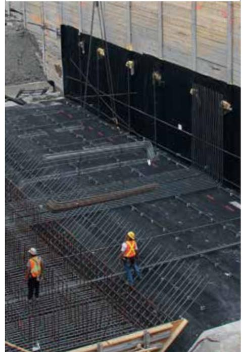
**PRECON** is a composite sheet membrane comprised of a non woven fabric and elastomeric membrane bonded to an exclusive plasmatic matrix. This product provides a permanent seal between the membrane and poured concrete wall or floor. It helps prevent moisture migration into the structure and improves resistance to termites, methane and radon gas. Make **PRECON** part of your next foundation waterproofing system.
