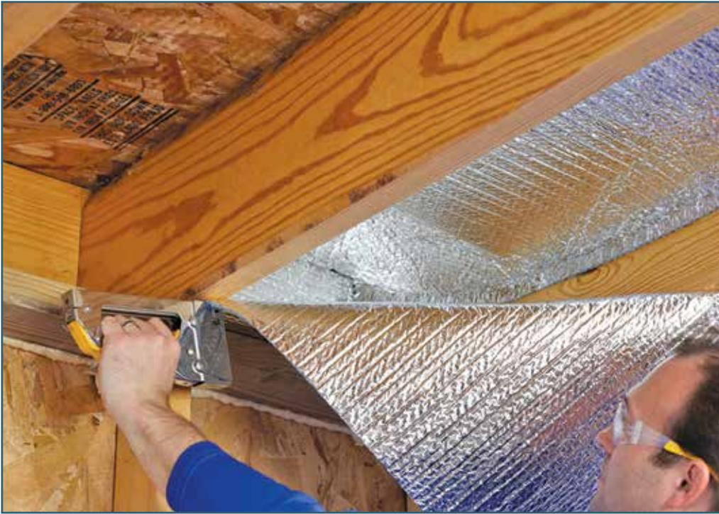
Figure 4 – Reflective insulation installation of a double-layer R-21 to a floor joist in crawl space.
