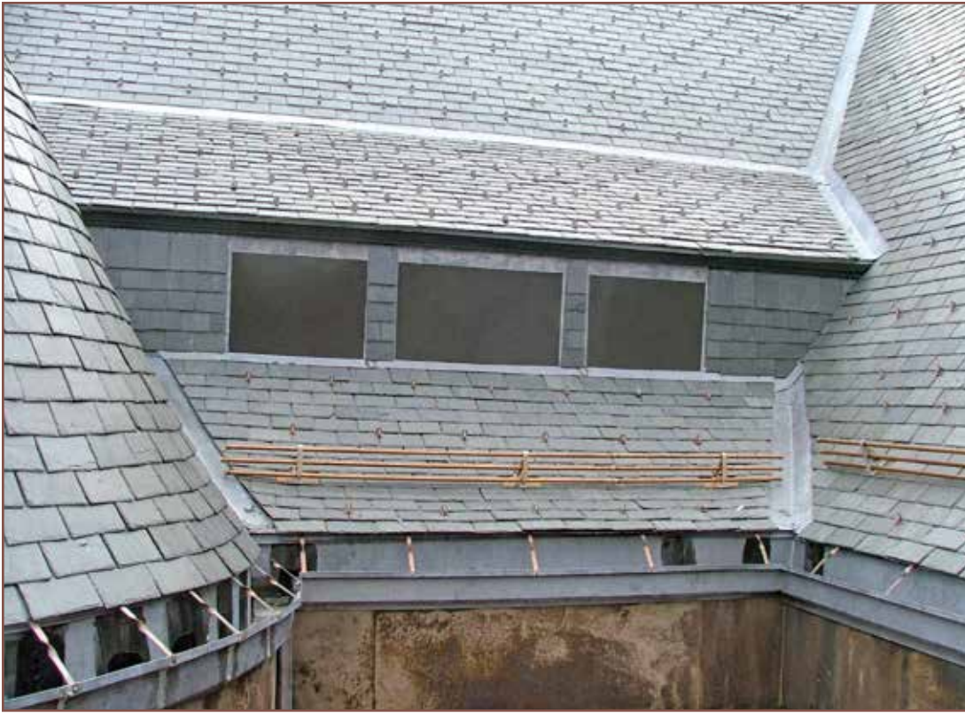
Figure 6 – Snow guard installation.
