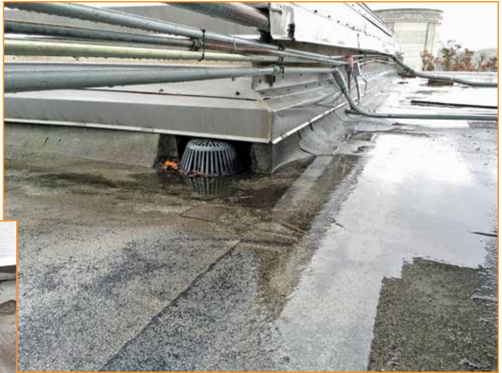
Figure 10 – Roof drain located inside an equipment curb.
