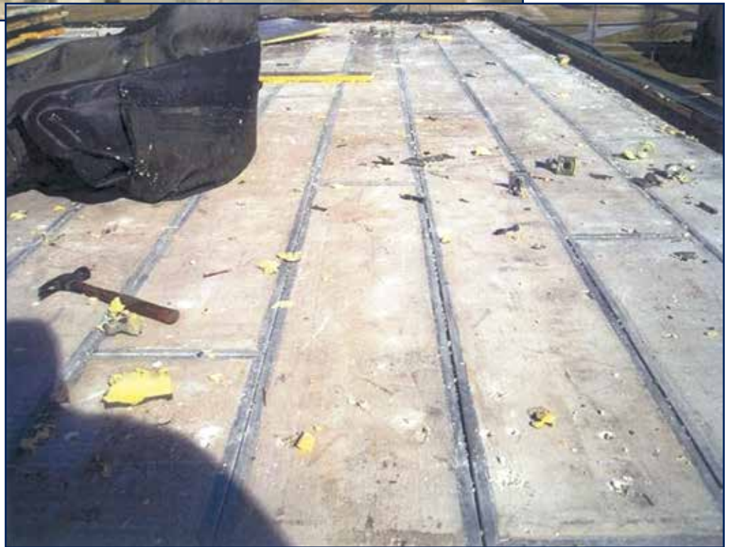
Figure 5 – This type of roof deck is obscure enough that some supply houses may not be aware of it. Accordingly, the particular roof-covering vendor should be consulted regarding its requirements for fastening to these planks. It would also be beneficial to work closely with a fastener vendor. (Image courtesy of Scott Hinesley.)
