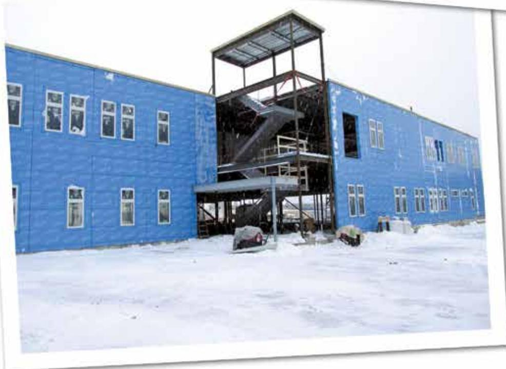
Figures 1 and 2 – Panelized walls were framed, insulated, sheathed, and fit with a vapor barrier and windows off-site. They were then transported to the jobsite, where they were raised in about three weeks. Almost as soon as the building was enclosed, heavy snow started falling. The siding and its accessories were installed in the spring. Photos by Ouellet Associates, Inc.
