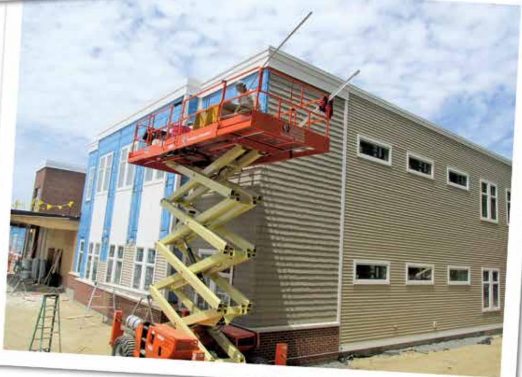
of design flexibility per the variety of profile, texture, and color options available on the prefabricated pieces. In addition, they were affordable. Ultimately, a mix of 4,600 square feet of modified polypropylene copolymer Perfection straight-edge shingles and 9,100 square feet of vinyl-lap siding were
