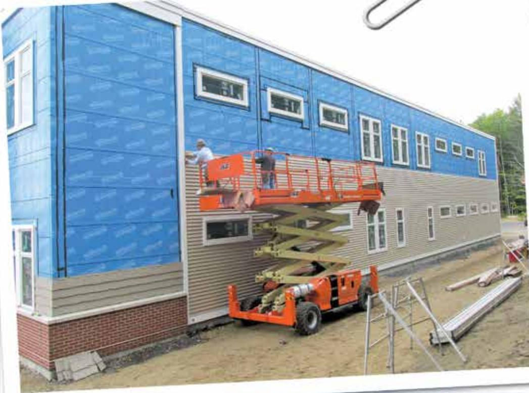
*Figures 3 and 4 – Ouellet Associates’s team installs vinyl siding in a woodgrain texture finish and 7-inch polymer staggered shingles onto a self-adhering air and moisture-barrier membrane. To complete all of the flashing, trim, trim panels, and siding, it took a crew of six to eight men approximately nine weeks.*
