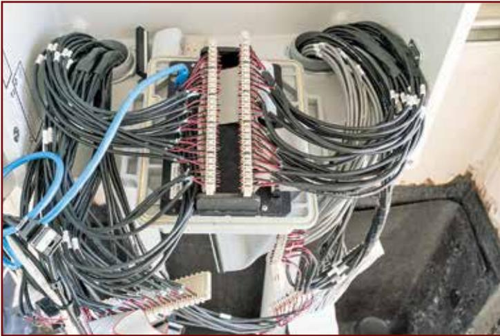
*Photo 2 – Wiring and scanning device utilized during construction of a leave-in-place electronic leak detection system.*
