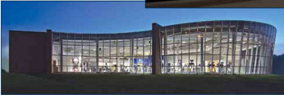
Figure 5 – Image of a large-scale installation of EC glazing at Butler County Health Care Center, David City, Nebraska. The application features a complex curved façade with glazing sloped outwards. The architects chose EC glazing because of the elegant solution to the heat and light control and the ability to maintain the views of nature on the campus for the patients in the rehabilitation center. Photo courtesy of Daubman Photography.
