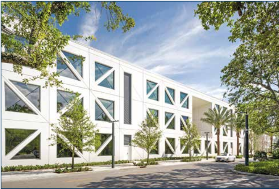
Figure 6 – Image of a large-scale installation of large, triangular-shaped EC glazing at the Frost School of Music, Miami, FL. Note the architecturally favored blue exterior reflected color. Photo courtesy of Moris Moreno.
