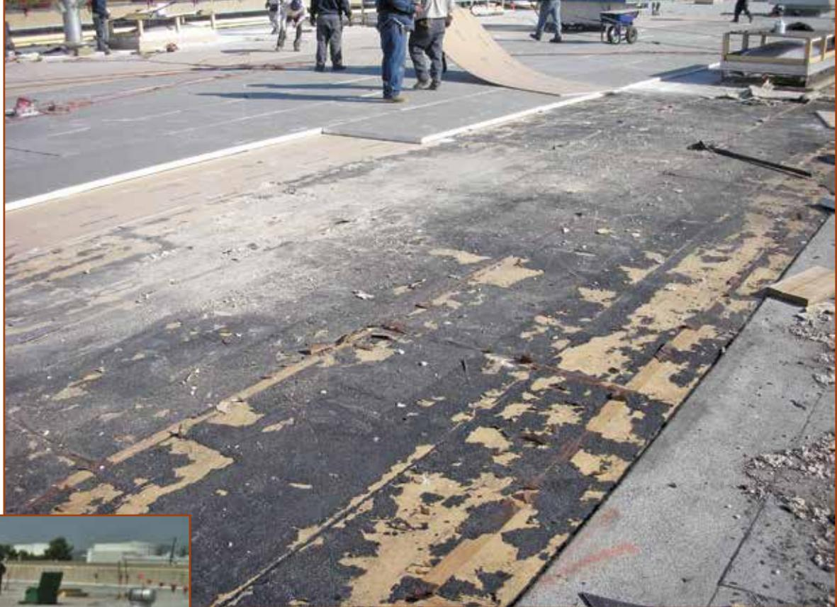
*Installation of roof covering over retrofitted Loadmaster roof deck.*
