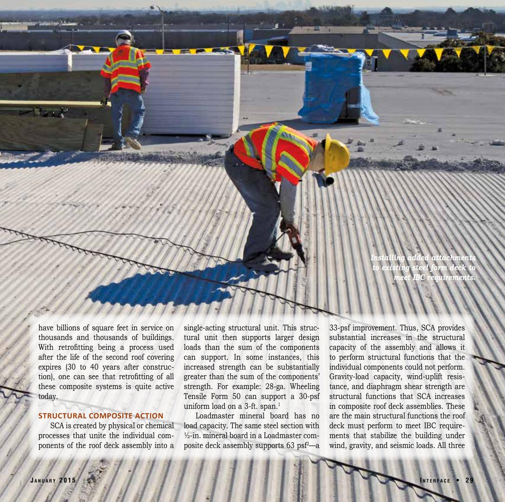
*Installing added attachments to existing steel form deck to meet IBC requirements.*
