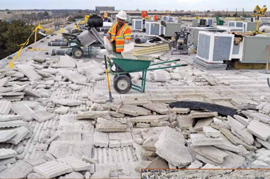
*Removal of wind-damaged LWIC from steel form deck.*
