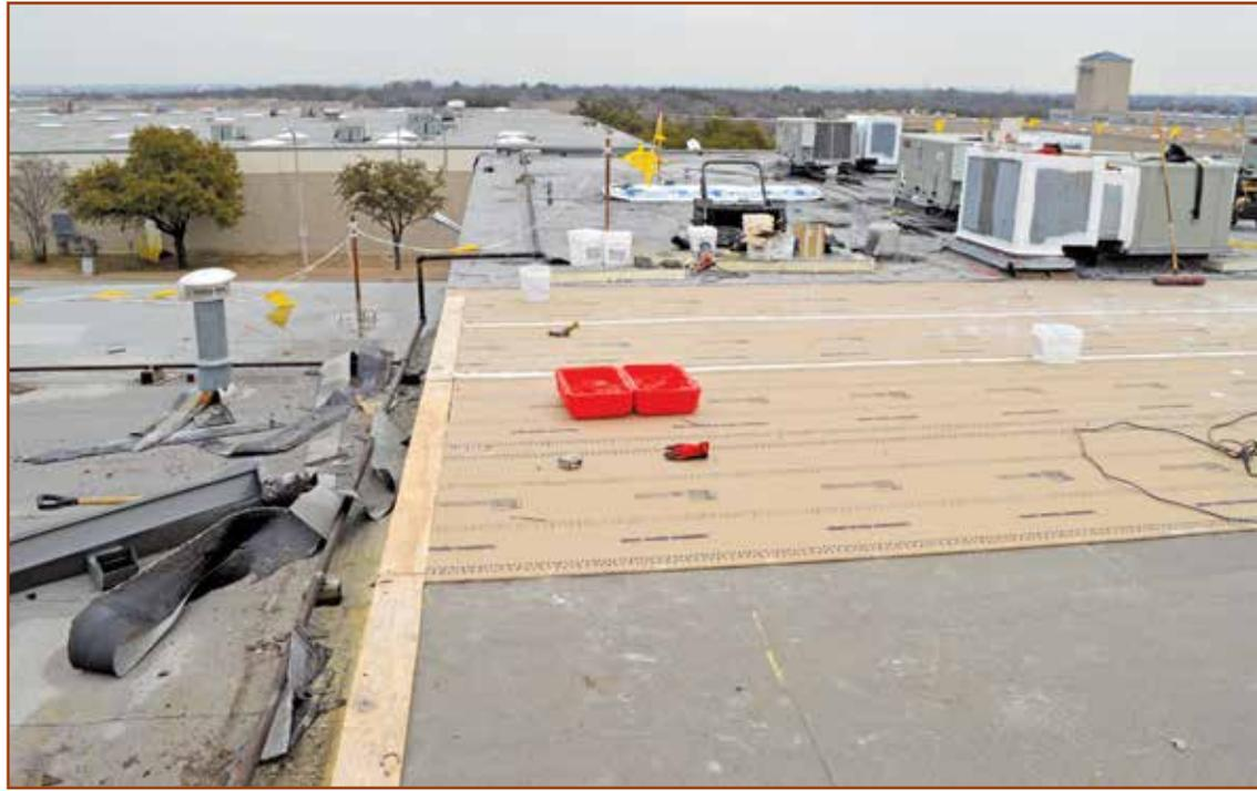
*Loadmaster composite components installed over existing steel form deck.*
