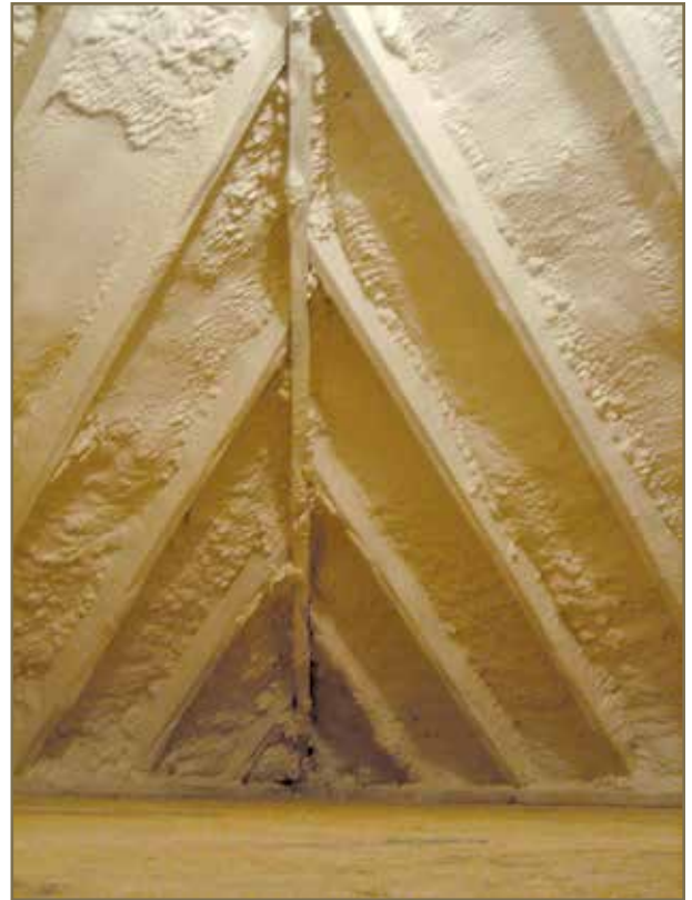
Photo 5 - Closed-cell SPF applied to the underside of a roof increases the racking strength.
