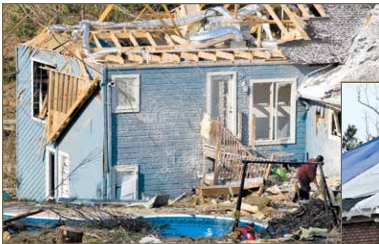
Photo 2 – Blown-off roof.
