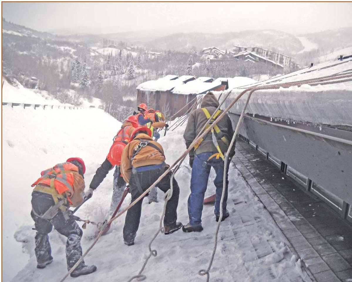
*Photo 1 – Workers remove snow from a building at the base of the Steamboat Springs, CO, ski area, where the average yearly snowfall is 480 inches and the elevation is 9,080 feet.*
