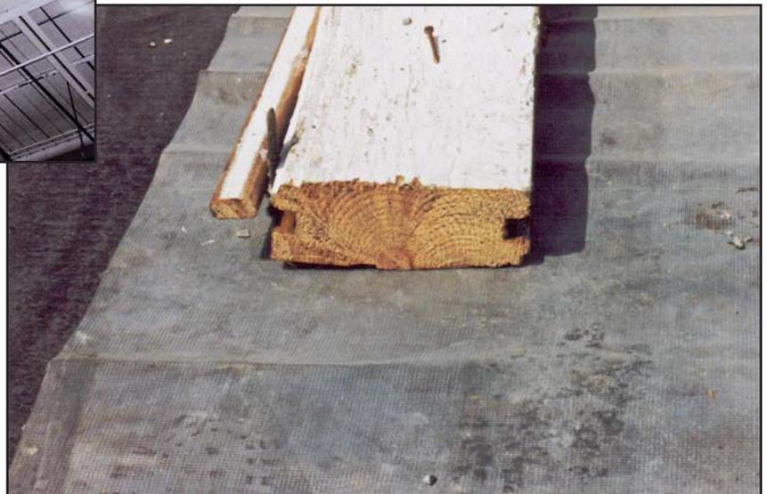
Figure 2 – Wood plank decks are commonly tongue and groove, but they can also be “splined” in the manner of heavier industrial wood floors.
