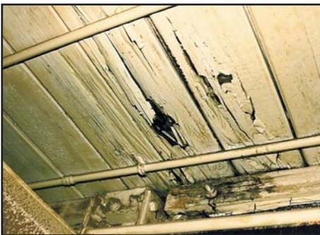
*Figure 5 – Inexcusable procrastination in addressing leaks can reduce a functional wood deck to a fall-through hazard. Underside paint can obscure this behavior during interior inspection, so be aware of this potential when preparing contract documents.*
