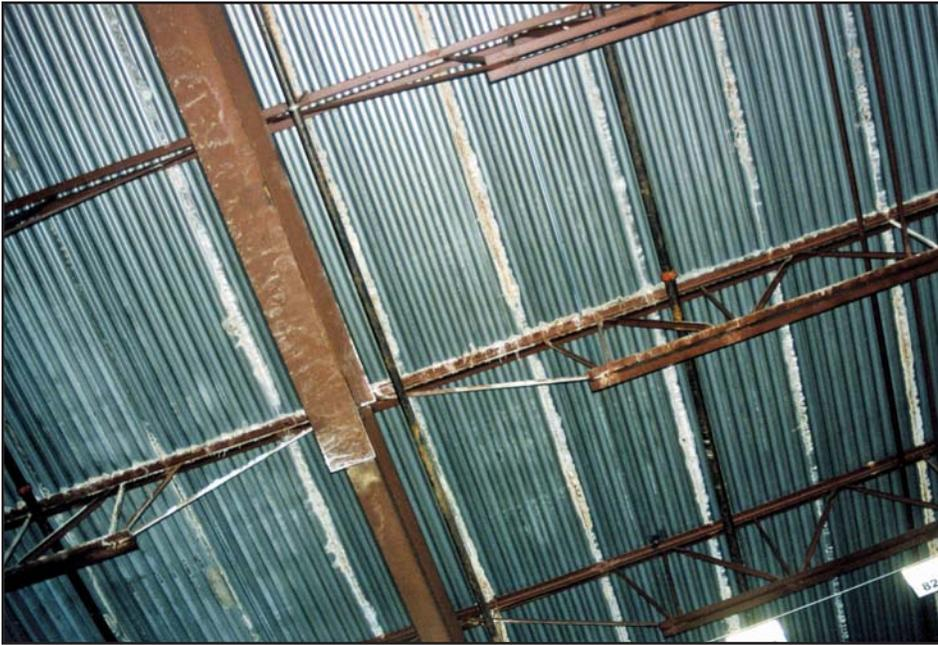
*Figure 3 — Often mistaken for a “metal deck,” LWIC is most commonly carried on a metal “formboard.” Modern iterations have slots at the bottom of the flutes/ribs to liberate construction water and induce continued drying. This image depicts an older version that predates slotted decks. The material emerging at formboard edges dates to the day it was installed and should not be confused with active leakage.*
