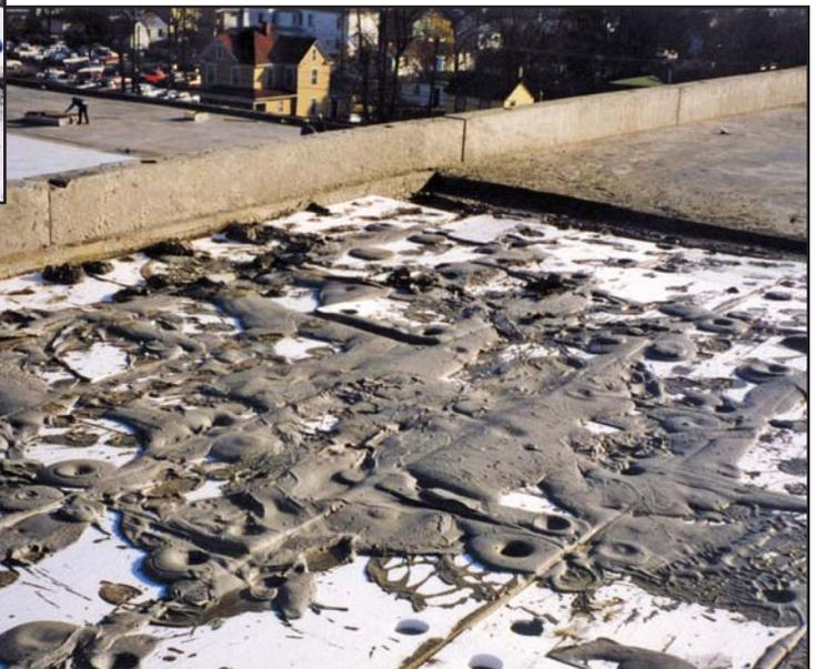
*Figures 1 and 2 — What may first appear to be a random mess is instead a quite viable roof deck system. Here, polystyrene boards are situated into wet LWIC. The polystyrene provides the bulk of the R-value, while holes and slots in the boards provide a “keying-in” of these materials.*
