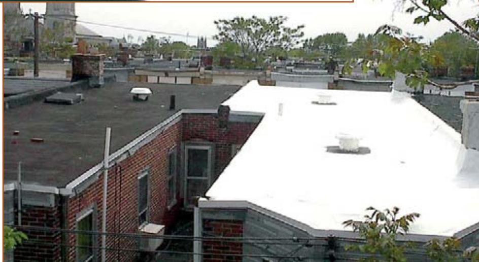
*Photo 2: Comparison of coated and uncoated roofs.*
