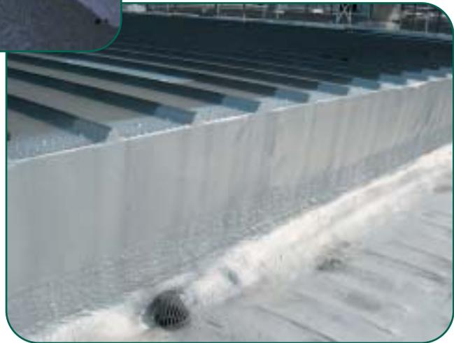
Figure 13 - SPF flashing, roof-to-wall.
