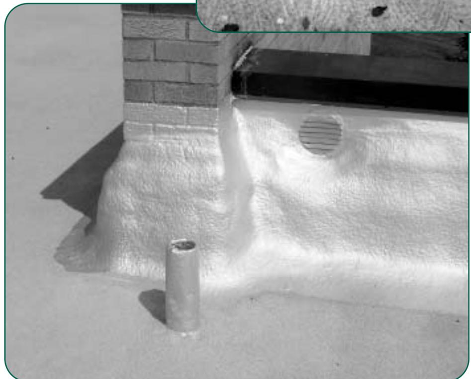
Figure 8 - SPF low wall flashing application.
