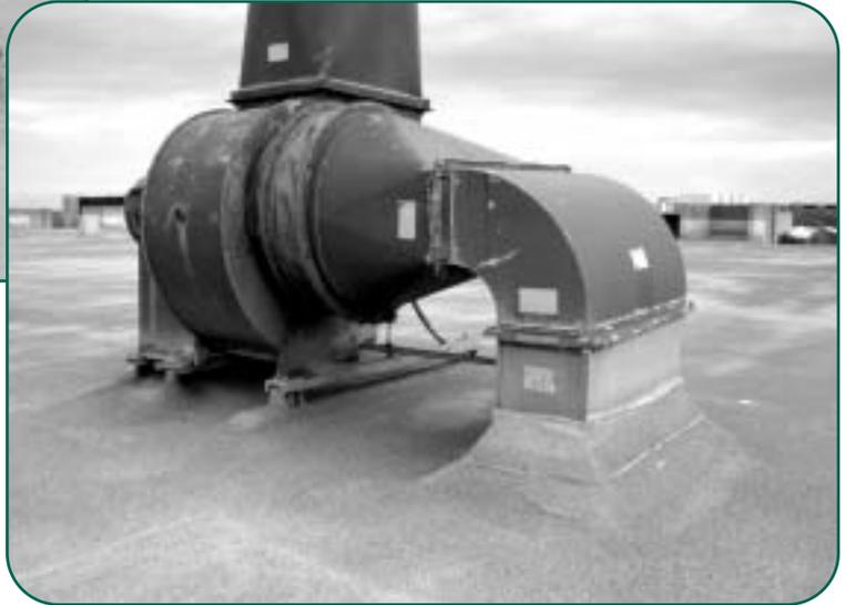
Figure 10 - Equipment support – low curb.
