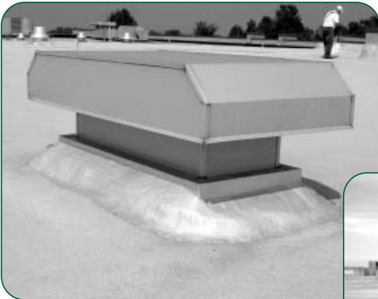
Figure 9 - Equipment support – high curb.
