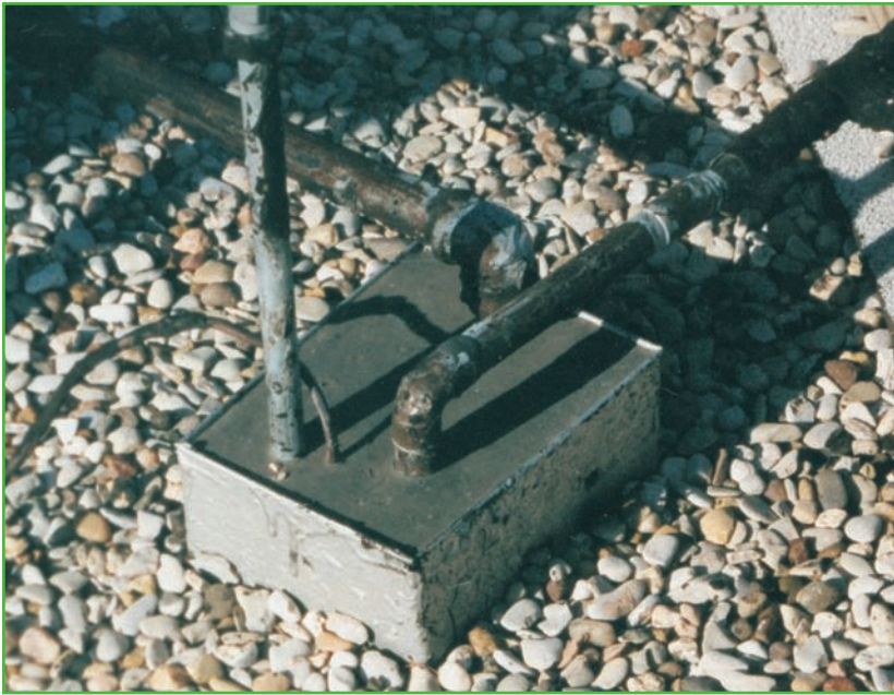
SPRI-approved pitch pan on EPDM.
