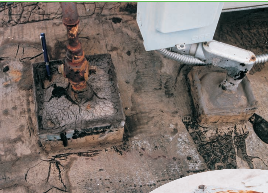
Above: NRCA pitch pans on a built-up roof.
