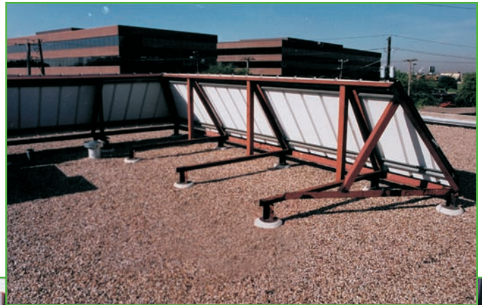
Right: Penetration seals on machinery screen over built-up roof.
