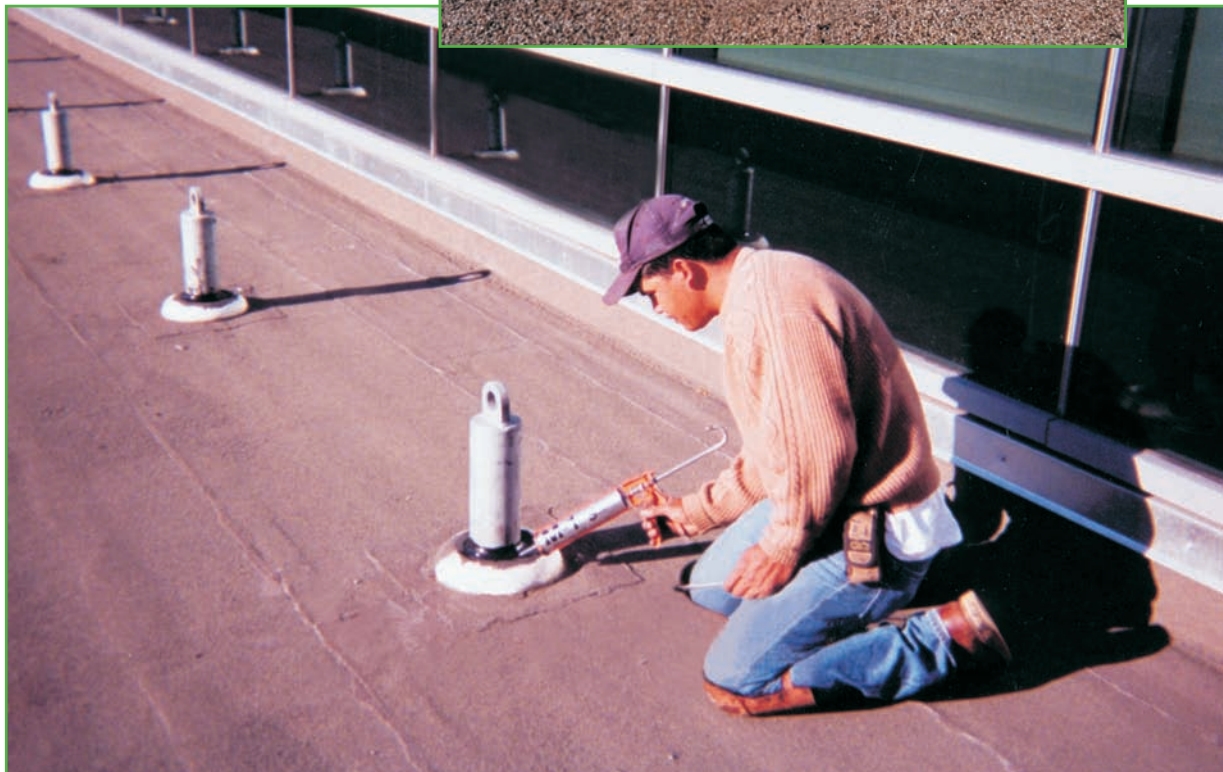
Right: Penetration seals on machinery screen over built-up roof.
