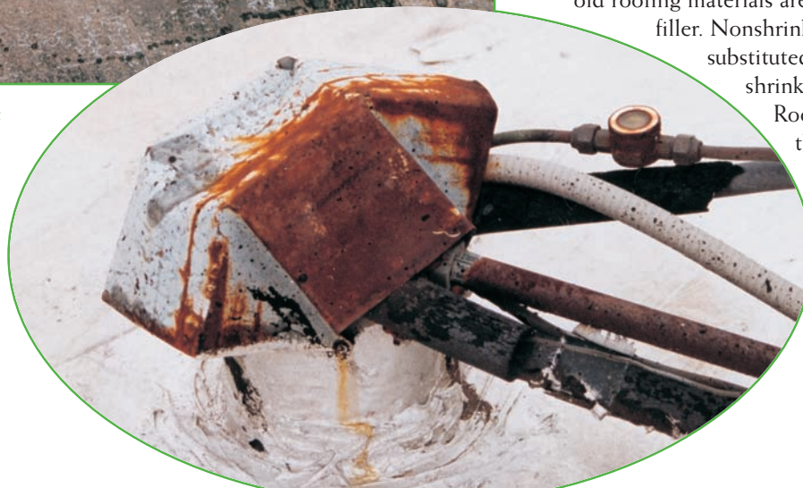
Above: NRCA pitch pans on a built-up roof.
