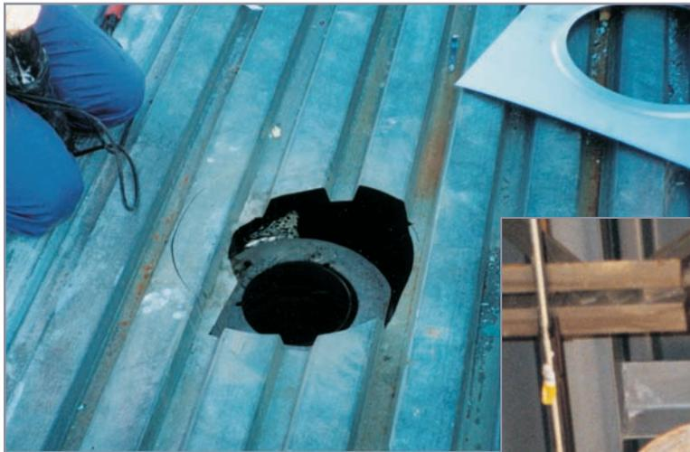
Figure 3—When two or more corrugations are cut from a fluted steel deck, things start getting soft quickly.
