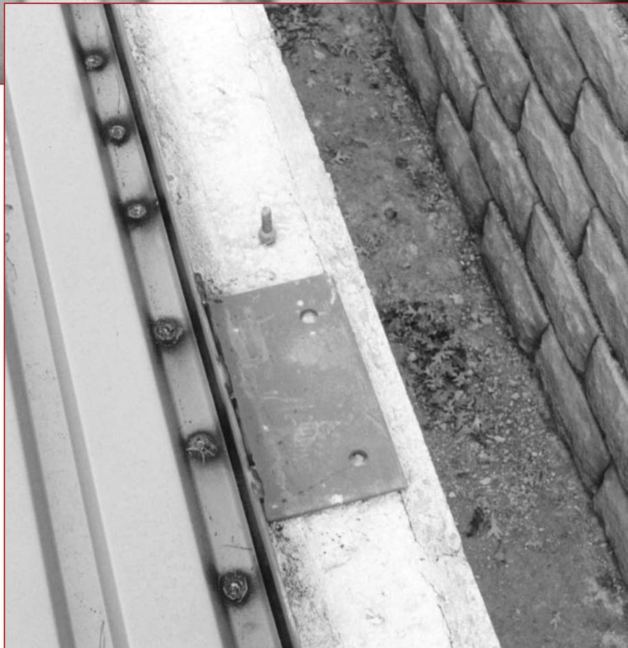
*Figure 9—Bond beams are the connecting link at the top of block and cavity wall construction. A number of framing and attachment methods may be encountered.*
