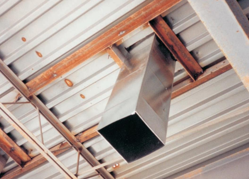
*Figure 4—An ideal arrangement of below-deck framing for a curbed mechanical unit. The curb that will eventually support the unit is not intended to serve as a structural element.*
