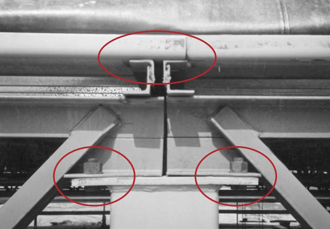
Figure 10—Expansion joints should be continuous through the edge carpentry and the wall construction, terminating at the footing. Rigid framing that traverses the opening violates the movement available.
