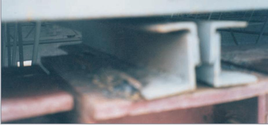
*Figure 5—Substandard weld length where a truss was merely tack-welded to a column capital. The entire flange of the truss should have been welded all around onto the bearing surface.*
