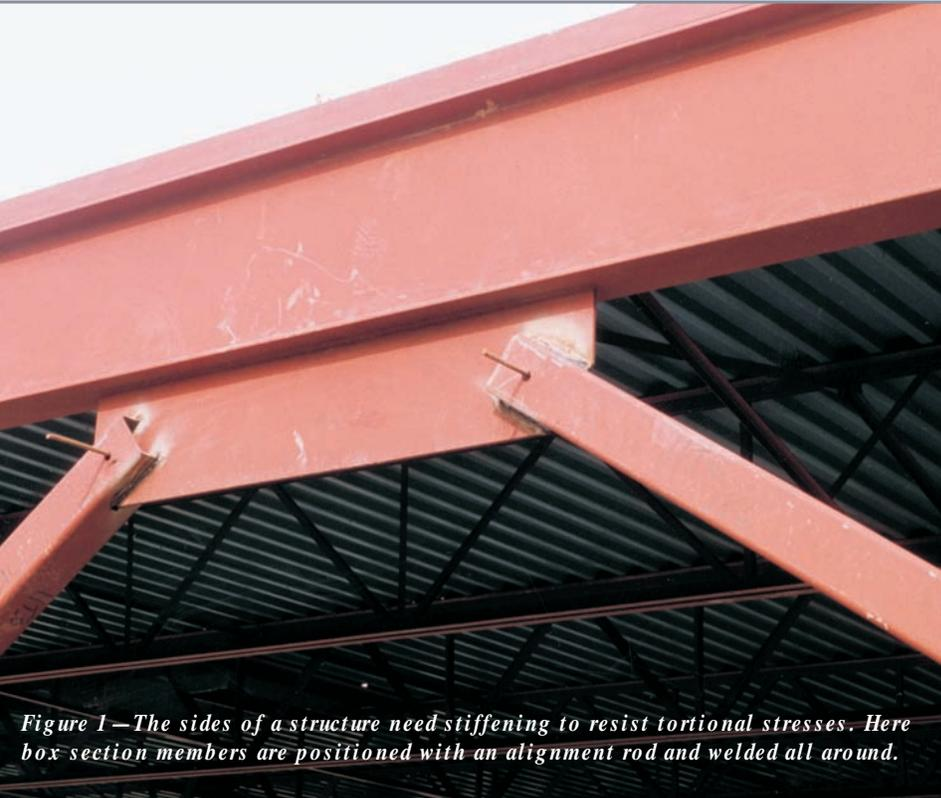
*Figure 1—The sides of a structure need stiffening to resist torsional stresses. Here box section members are positioned with an alignment rod and welded all around.*
