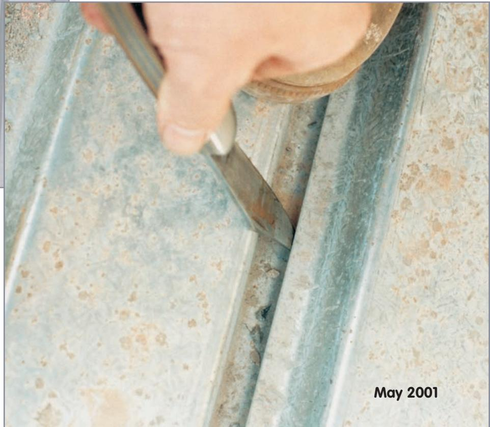
*Right: Figure 7—A steel deck, when properly fastened, will serve as a horizontal shear diaphragm. However, the diaphragm is not functional until the side lap stitching screws are installed.*
