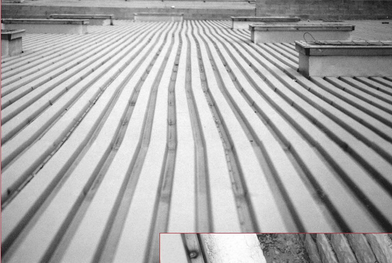
*Figure 8—Meandering deck sheets (above) are a real frustration for the roofing contractor. Deck sheets should align to within 1/4-inch per hundred feet of length.*
