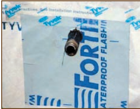
Figure 3: Penetration integrated into drainage plane.
