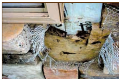
Figure 2: The consequences of reverse lapping.
