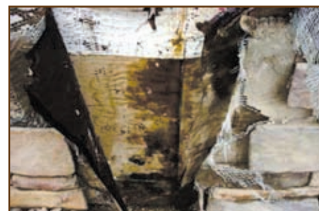
Figure 2: The consequences of reverse lapping.
