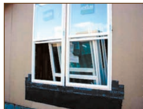
Figure 1: Examples of precut sections of building paper under windows to ensure proper lapping.
