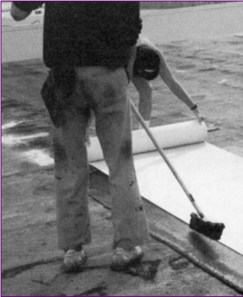
Fig. 2: “Stitchbonded” polyester fabric being installed. Courtesy RSI, May 1991.
