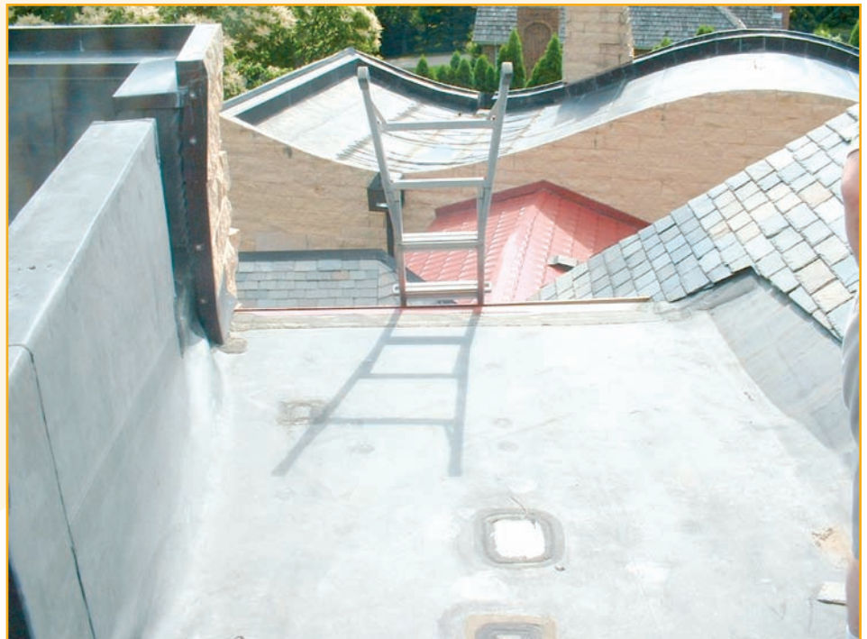
Photo 4. The roofing on this contemporary home has four different roof structures, each with different roofing and cladding systems. A roof consultant’s involvement may have increased efficiency for the design team during design and construction administration phases.
